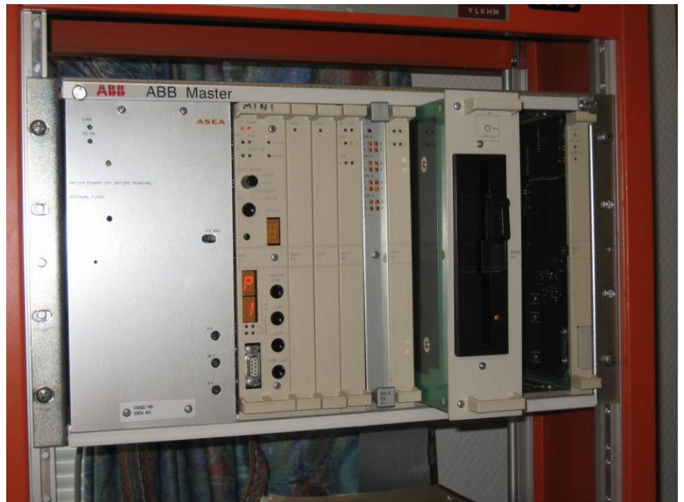
Figure 14 Remove the old DSMD 113 unit from the MasterView rack.
