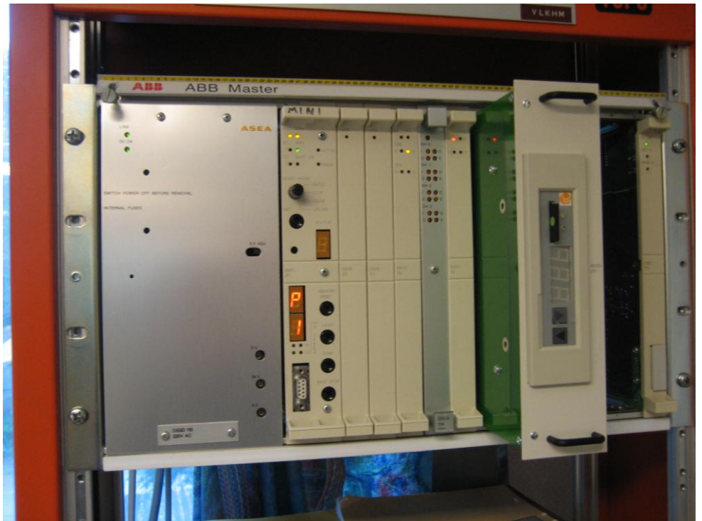
Figure 15 Insert the new NDDD 001 circuit board in the MasterView rack.
