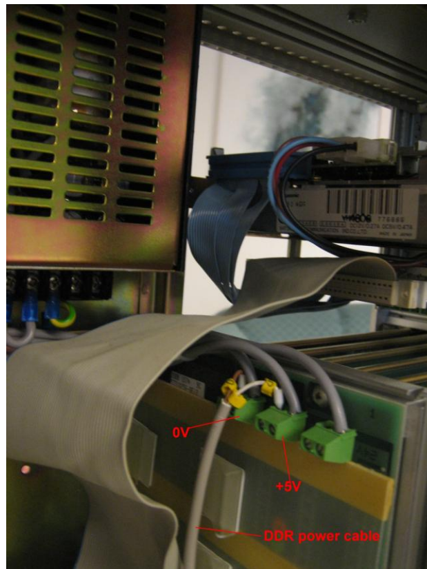
Figure 17 The 0V and +5V power screw terminals in the MasterView cabinet.
